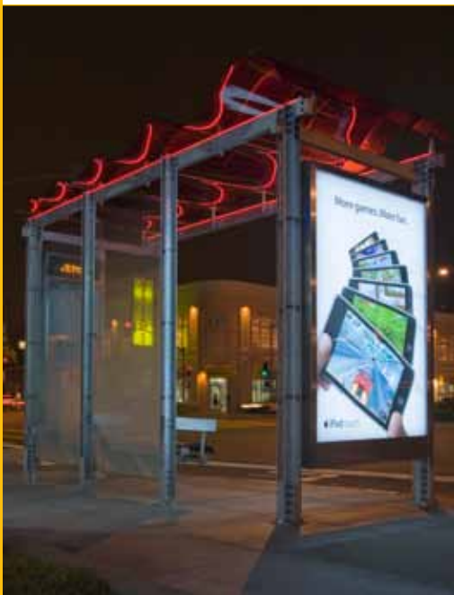
San Francisco MTA Transit Shelter at night
